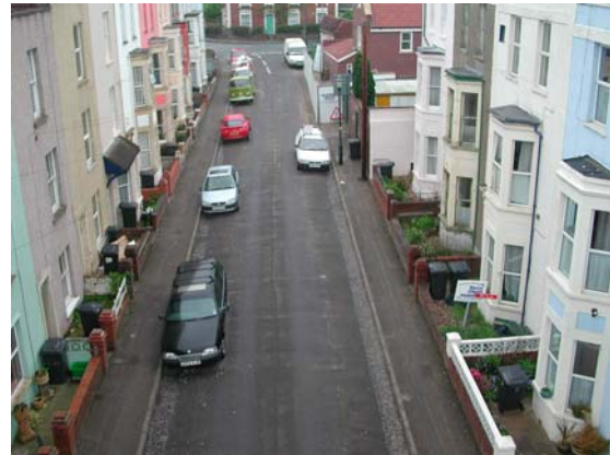
Fig. 1: Milford Street prior to Home Zone
