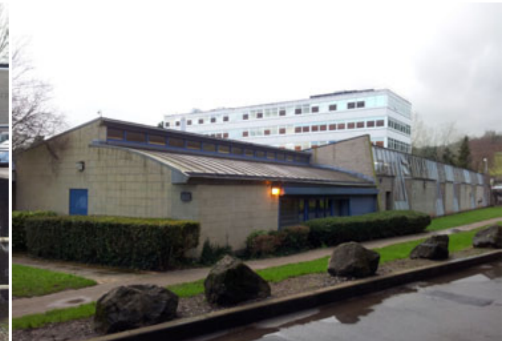
View looking up Kennel Lodge Road. Proposed site with existing G Block is seen on the left. The 5 storey B Block building can be seen behind.
