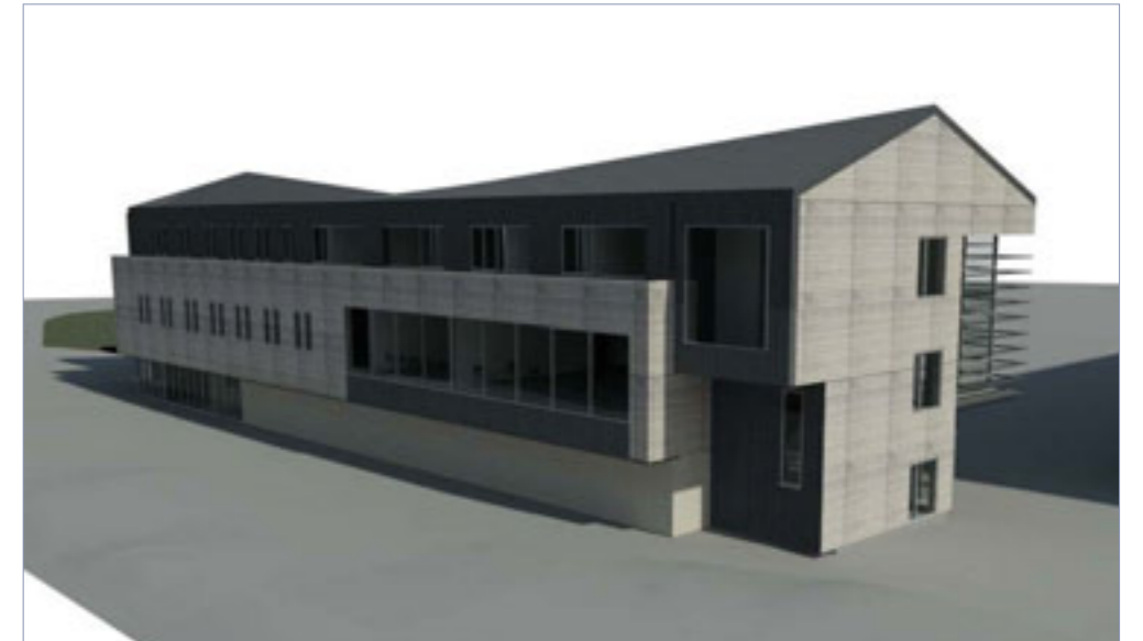
VERSION C - BOWED ROOF PROPOSAL WITH FIRST FLOOR PROJECTION. METAL CLADDING AT TOP FLOOR STEPPED BACK FROM THE TIMBER CLADDING ON THE NORTH FACADE.
