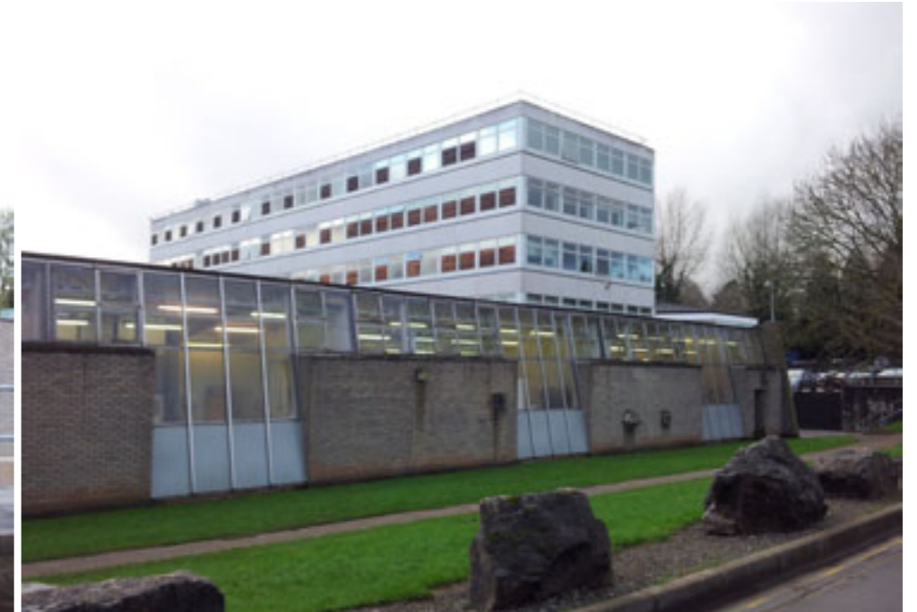
View from Kennel Lodge Road looking south west towards the proposed site. The existing G Block building is in the foreground, with the larger B block in the background. Note the road rises approx. 1.5m from east to west along the proposed site frontage.
