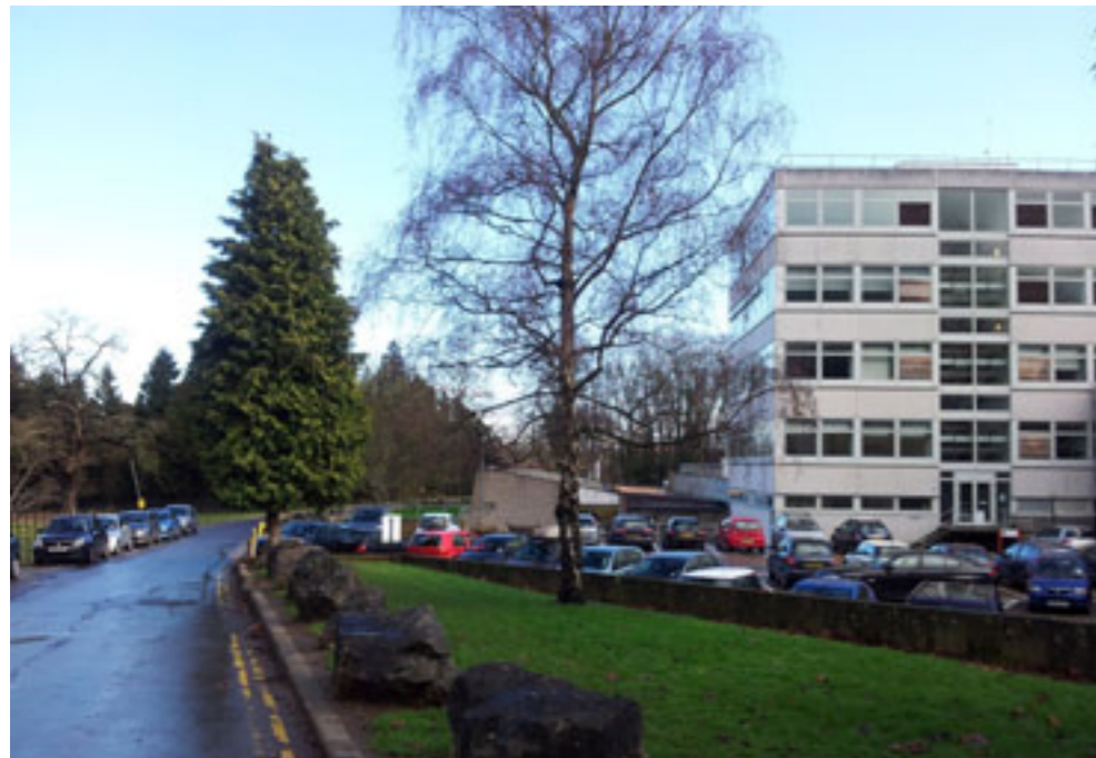
View looking down Kennel Lodge Road with proposed site directly in front and to the side of the 5 storey B Block building. Note lack of footpath along the road.
