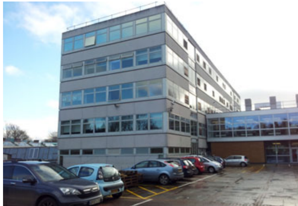
View of existing main campus entrance to A Block. The entrance approach is dominated by car parking, presenting an unattractive frontage. The proposed scheme will improve this important external space, creating a new pedestrian area, cycle parking and reduced car parking.
