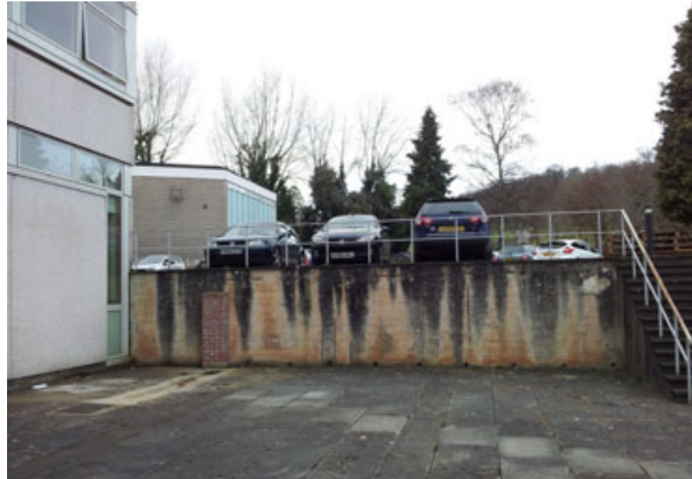
View of the existing concrete pit to the west of G block. Note the level difference of approximately 2.2m up to the car park behind.
