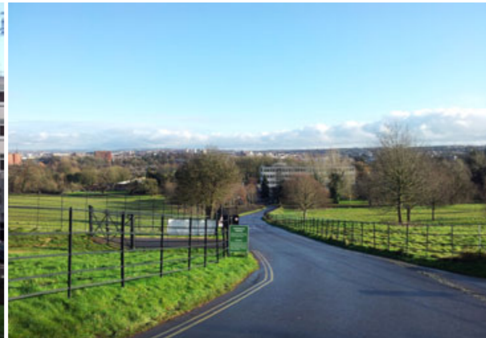
View looking down Kennel Lodge Road from Ashton Court Estate. The existing campus sits at the bottom of the hill within mature trees. The 5 storey B block building can be seen through the trees.
